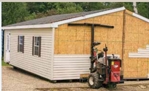
Moving a modular garage into position
