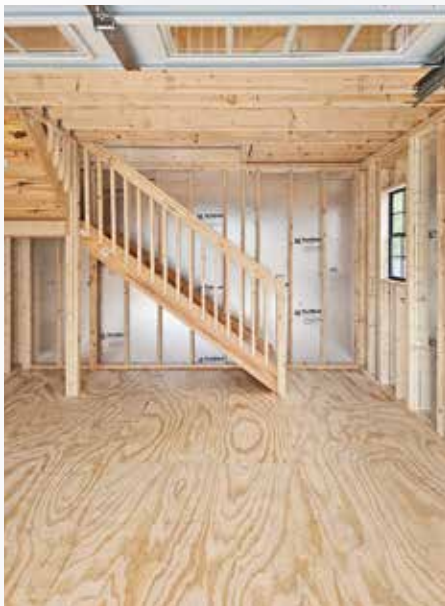
Inside View Facing in from Garage Door
