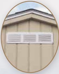
Painted siding gable vent
