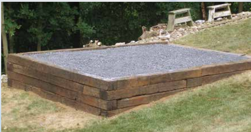
Shed pad with railroad tie wood retaining wall, built on a hillside.
