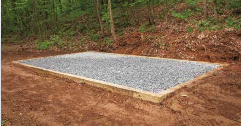
Basic shed pad with pressure-treated wood framing.
