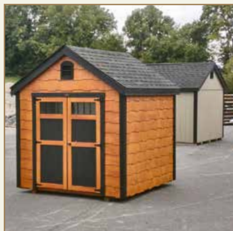
Stained or painted LP shake siding
