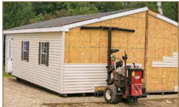
Moving a modular garage into position
