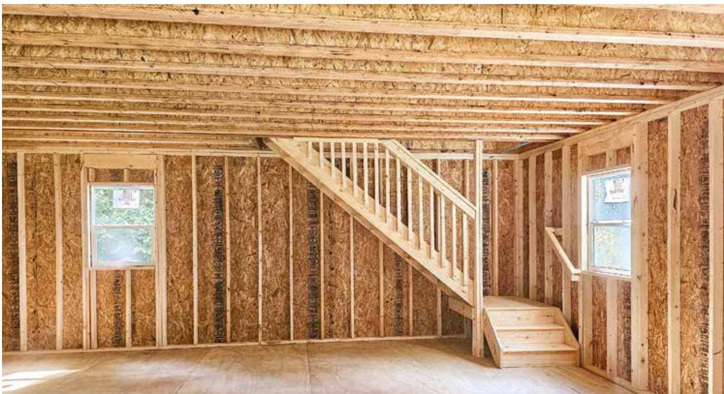
Inside First Floor Facing in from Garage Doors
