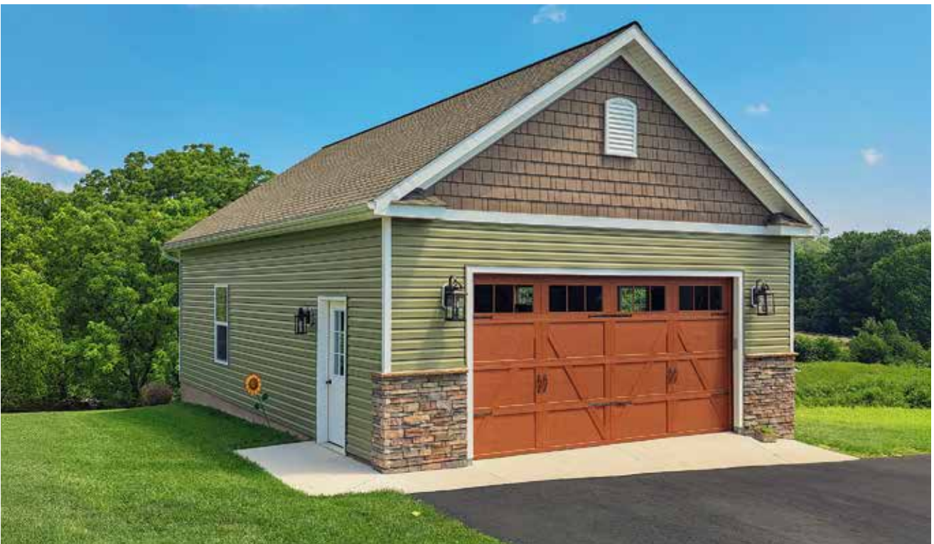
G60 | 24x28 with Attic Trusses Custom colors with stone front and cedar impression shakes on gable
