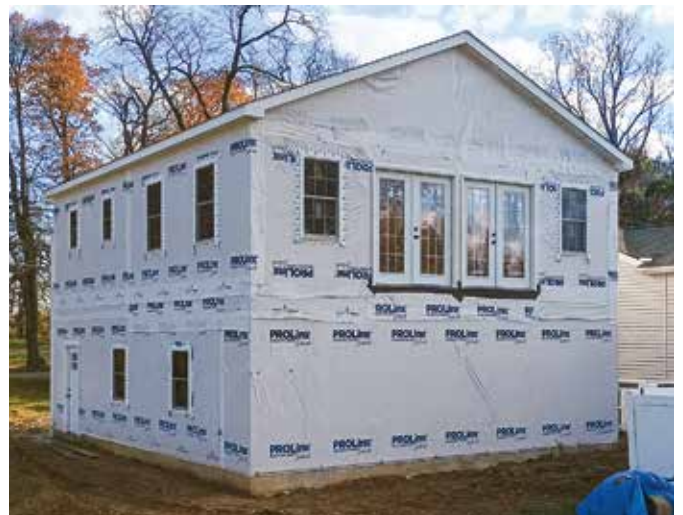
G81 | Full 2 Story in Progress
