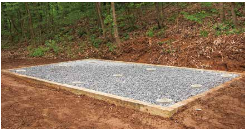
10x12 shed pad with concrete pillars, rarely needed.
