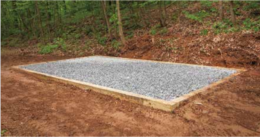
Basic shed pad with pressure-treated wood framing.
