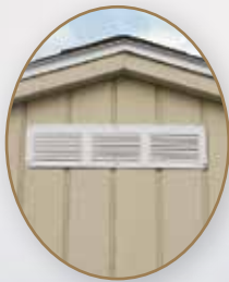
Painted siding gable vent
