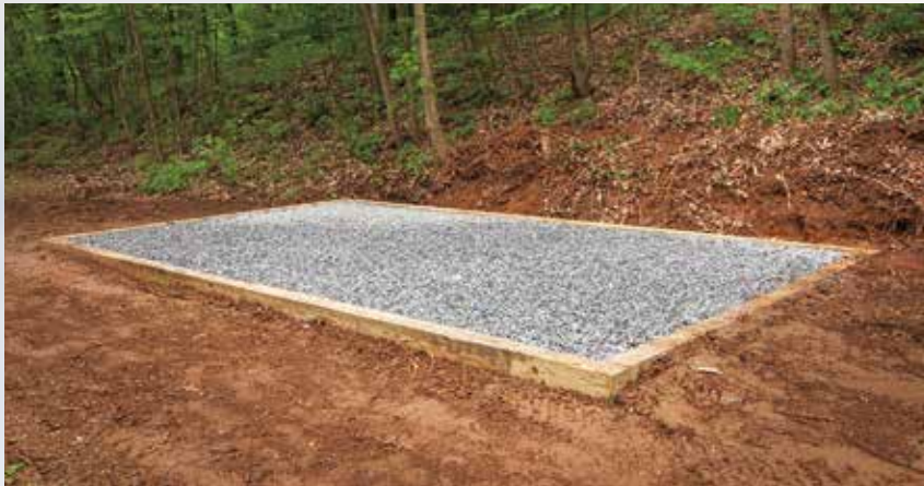
Basic shed pad with pressure-treated wood framing.
