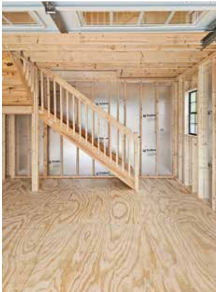
Inside View Facing in from Garage Door
